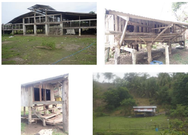
Figure 4. Housing management: Over pole type of housing; East – west house orientation; and Galvanized house roofing.
